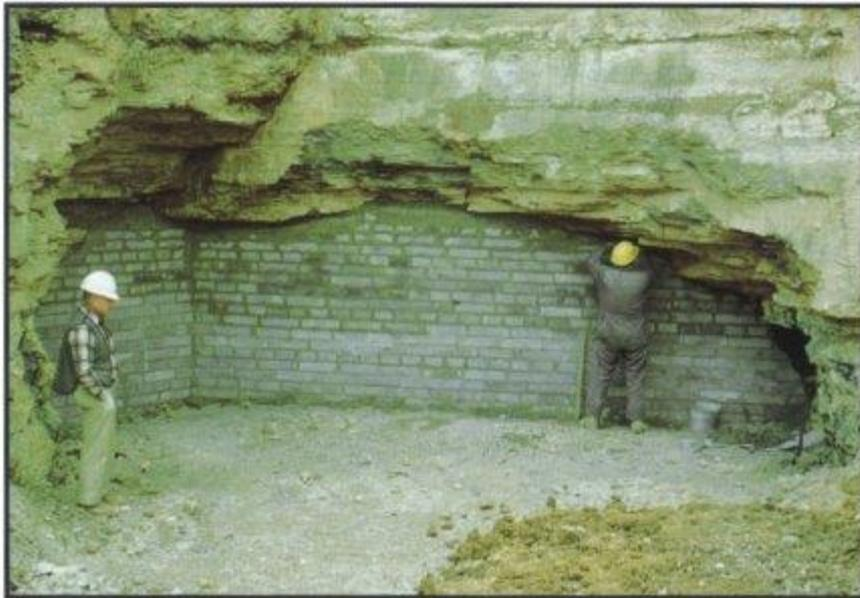
**A concrete block dry seal placed at an abandoned mine land reclamation project in West Virginia.**
